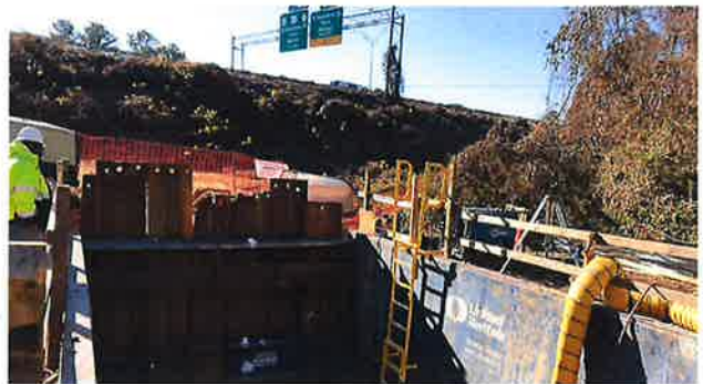
S. Saunders Sanitary Sewer Improvements, Raleigh, NC
